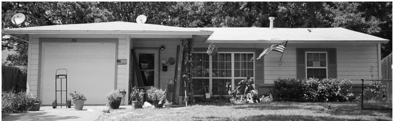
Ruth Hyde Paine’s House at 2115 West 5 th Street, Irving, Texas On November 3, 2013 the house became the Ruth Paine House Museum.
